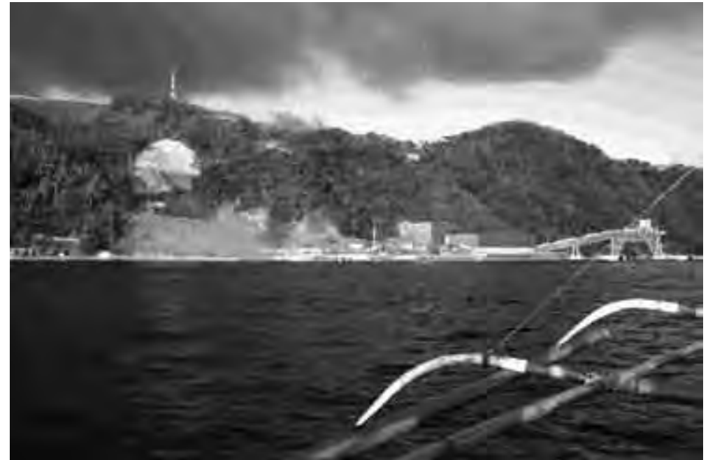
A landslide at the RapuRapu mine: part of the extensive damage that occurred to buildings and the environment after the November 2006 typhoon.
