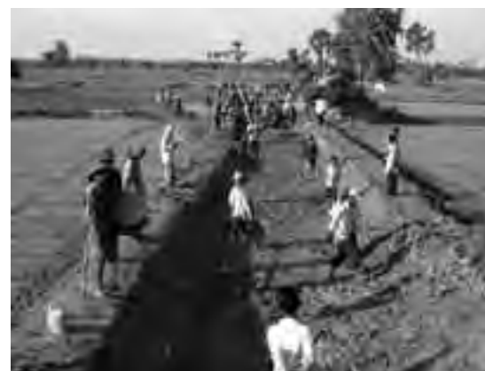
Canal rehabilitation in Cambodia. Source: Development Partnership in Action
